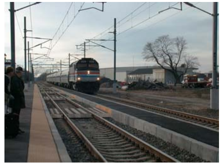
This is a picture of the train coming in to Kingston station. Note: there are wires on top of it even though the train is diesel. These wires are being used for Acela Regional.
